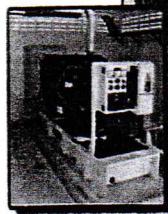
FG WILSON ▶ P1500E (1500kVA) ▶ P1500E (1500kVA) ▶ P1500E (1500kVA) All 12 Sets
